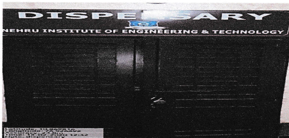
Dispensary at Nehru Institute of Engineering and Technology
